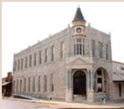
First National Bank, Stephenville, TX. Photos: NPS files
