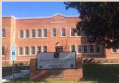
Harnett County Training School, Dunn, NC Photos: NPS files
